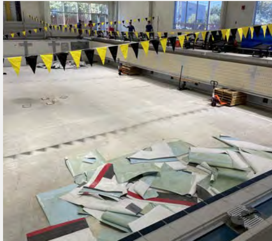
The FMH Competition Pool during the relining process in 2023.
